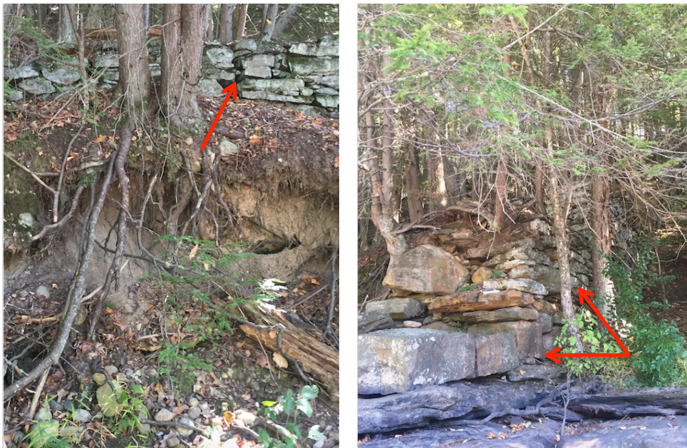
Figure 3.12: Remnant dam along the Salmon River. Arrows point to dam structure embedded in the bank.
