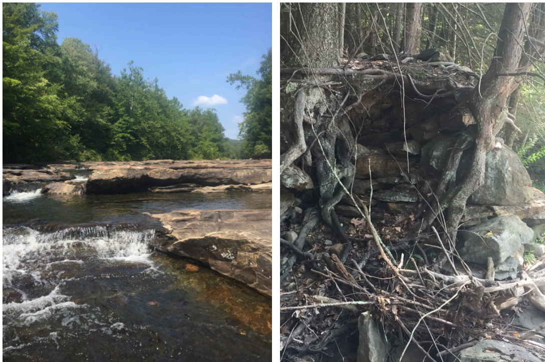
Figure 5.11: Downstream Salmon River view looking upstream and left bank dam remnants with displaying no visible fine-grained sediment deposits.
