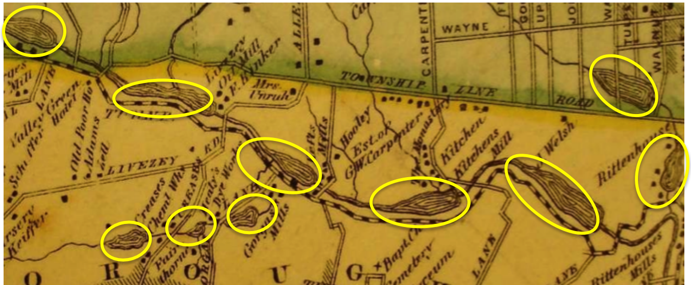
Figure 3.3: Historic map of dam locations in Lancaster, County. Dam locations are circled. Source: Franklin and Marshall College.
