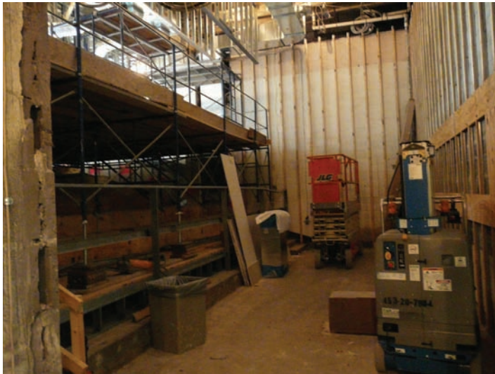
Bill 106 temporary construction floor and mechanical lift, as viewed from the front of the room, Summer 2008
