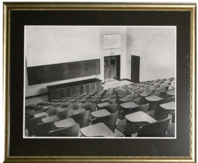
Original Bill 106 before renovation.
