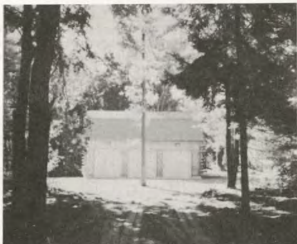
Built in 1990 near Gallows Lane and Buck Lodge, this garage houses Arboretum maintenance equipment. Tract 1. (G. Dreyer)
