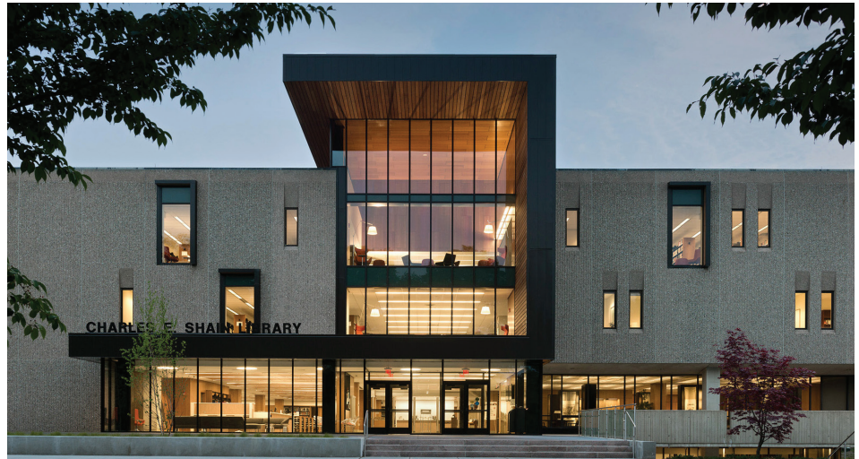
IN NAMING SHAIN AS A NEW LANDMARK LIBRARY, JUDGES FROM LIBRARY JOURNAL PRAISED THE CREATIVITY, INNOVATION AND RESOURCEFULNESS OF THE RENOVATION DESIGN.
