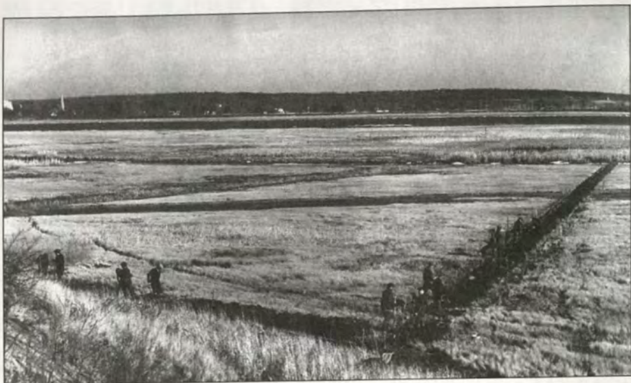
Fig.3 Many miles of mosquito ditches were hand-dug during the Great Depression. (DEP)
