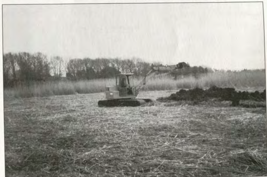
Fig. 10 A low-ground pressure excavator digging a creek during the restoration of a buried marsh. (R. Rozsa)
