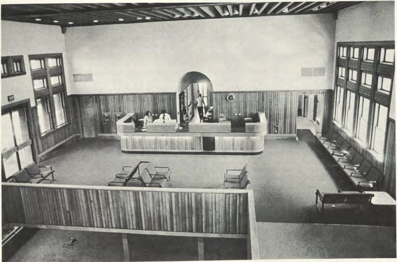
After: New coat of paint, relocated ticket counter, and split-level waiting area with upholstered seating.
