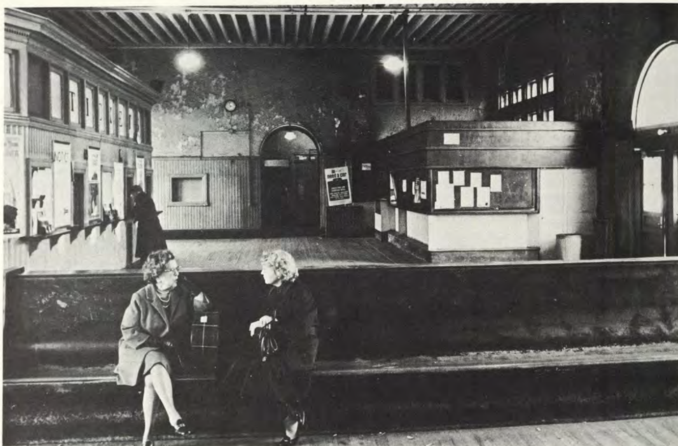
Before: Waiting room dominated by grime, peeling paint and uncomfortable wooden benches.
