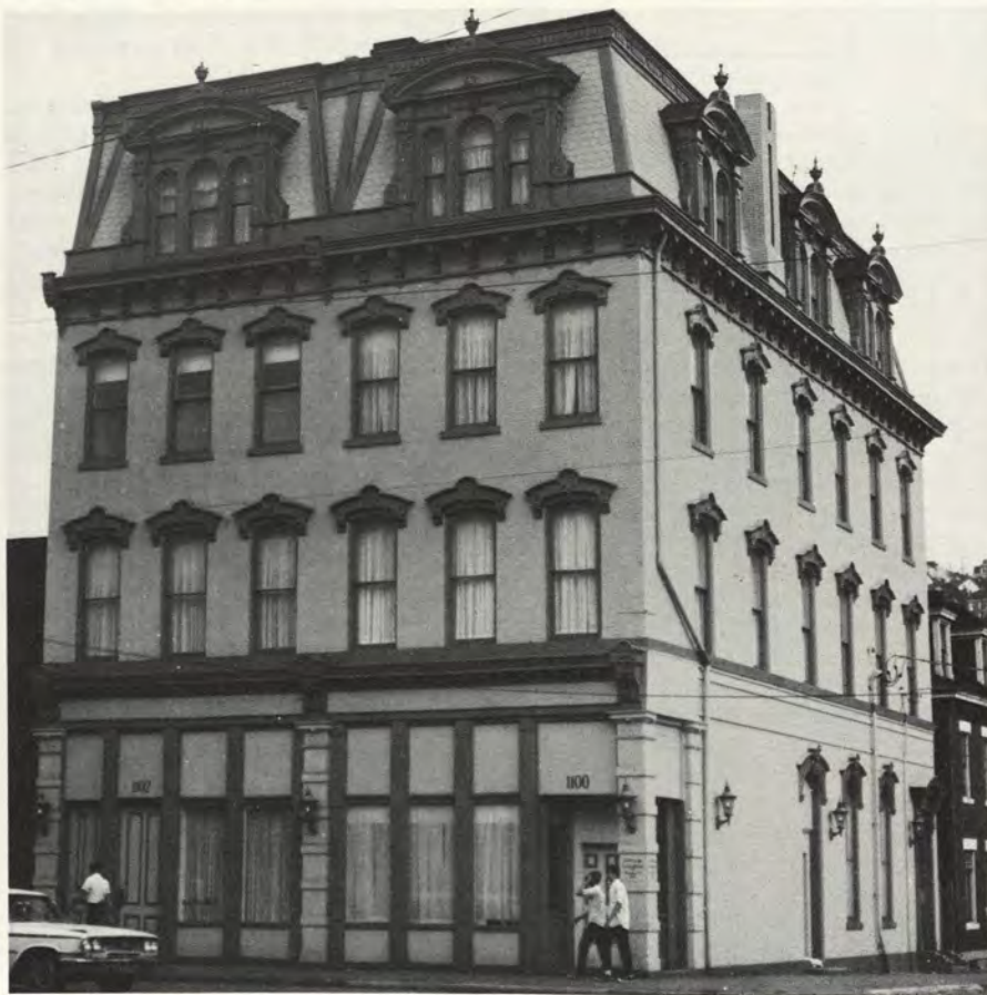
Restoration on the South Side (left).
