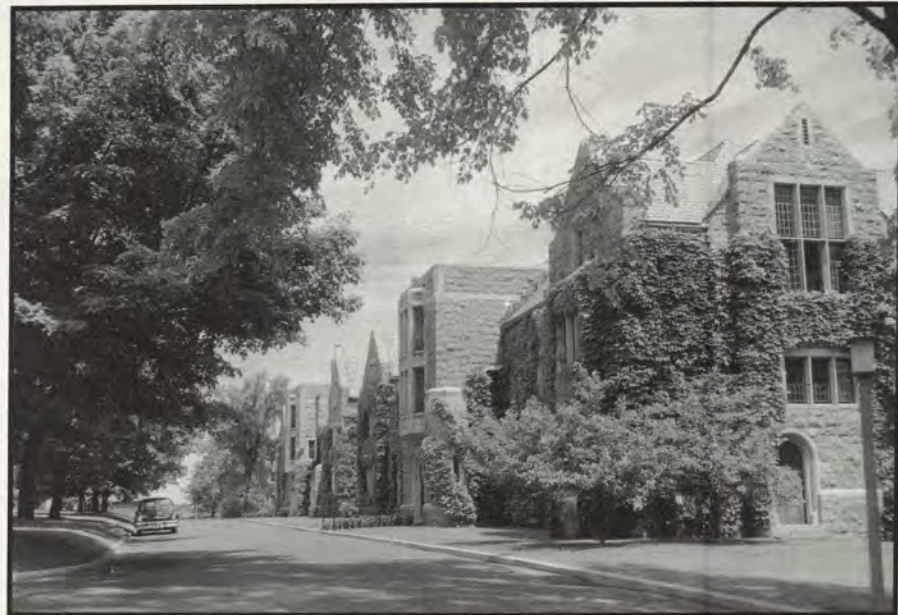
Plant House and Branford House dormitories, which were built in 1914. The ivy was taken down in the mid-1970s.
