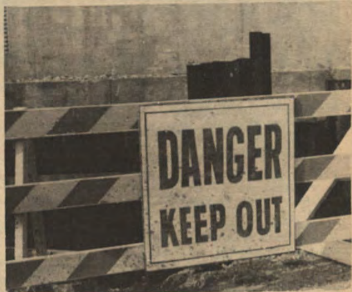
Bridge building carries on.
