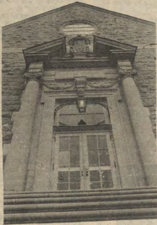
Waiting for renovation - Palmer Library
