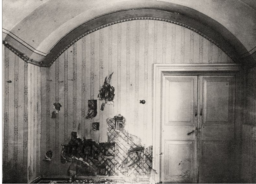
Fig. 1. File:Ipatiev House – Cellar room.jpg . Available from: Wikimedia Commons, http://commons.wikimedia.org/wiki/File:Ipatiev_House - Cellar room.jpg
