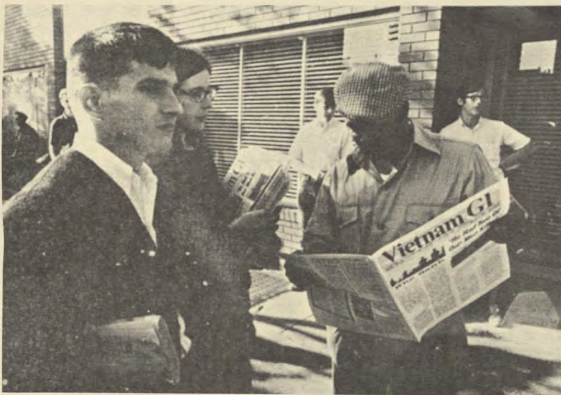
Early morning work at the Induction Center
