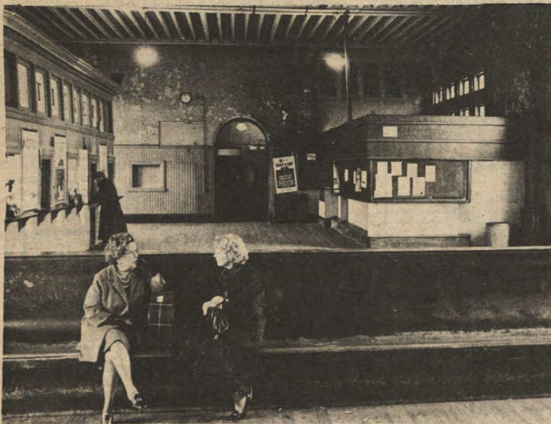
YOUR BASIC 'BEFORE' PICTURE: Severe dilapidation of Union Station before renovation is evident in this view, which shows main entrance at far right. Straight ahead is area where present ticket counter sits. Note peeling paint and cracked plaster on far wall. Photo courtesy the New London Day.
