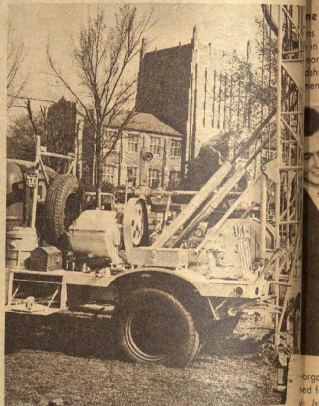
This portable drilling unit has been set up on the Tulsa University Campus to provide engineering students with a first-hand demonstration of drilling techniques. No oil has been struck as yet, but in this petroleum-rich area anything can happen, and the engineers may find that they have a gusher on their hands before long.
