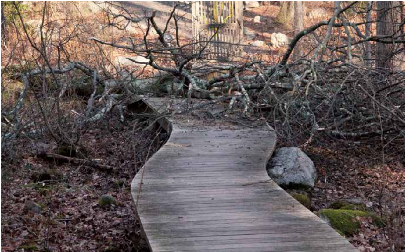
The board walk between the wildflower and conifer collections was damaged by a large falling tree.
