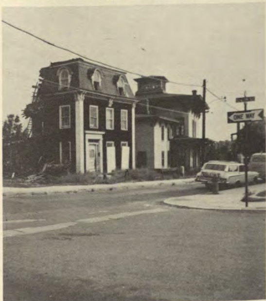
MAIN STREET homes are demolished to make way for redevelopment.
