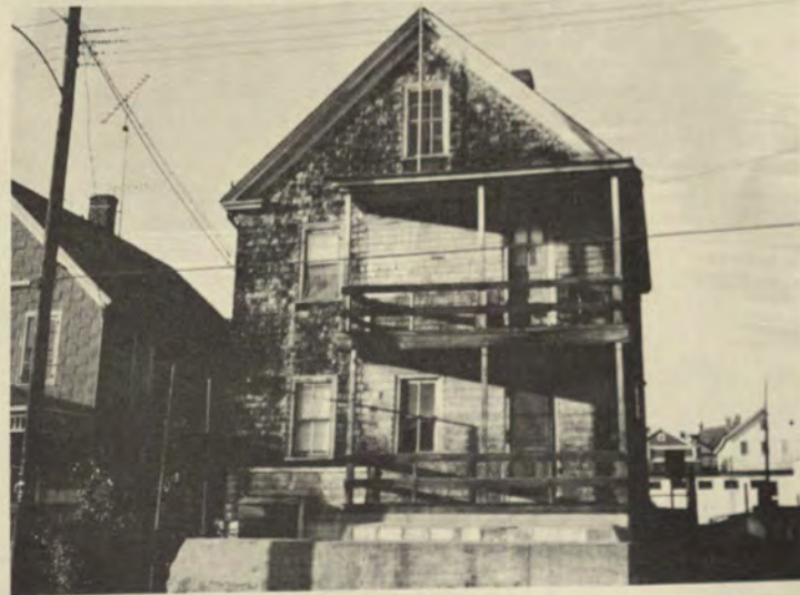
TYPICAL of the present Shaw Cove Area is this slum housing which redevelopment officials hope to eliminate.
