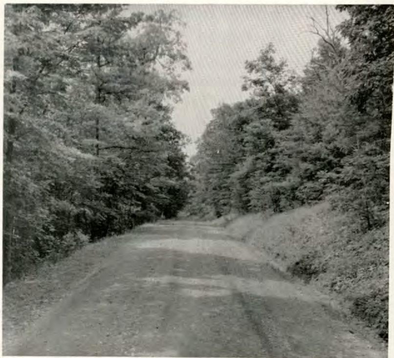
Fig. 1. A road on the George Washington National Forest two years after spraying in 1957. Shelf construction along a slope, with bank on one side and drop-off on the other, is typical of many forest roads. With selective oil-basal spraying, the bank remains stabilized under herbaceous cover.
