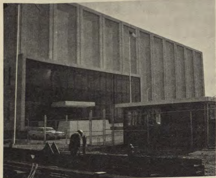
A recently completed building at the Millstone Power Station.
