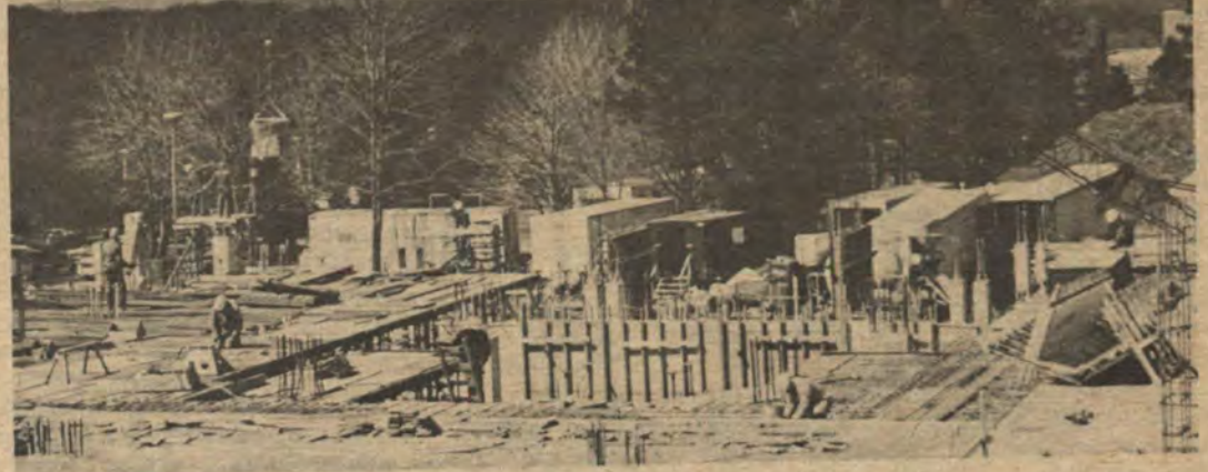
Lowering the boom on new library construction
