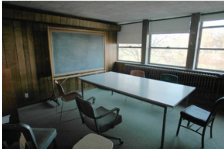
Bill Hall Room 409 before renovation in April 2007
