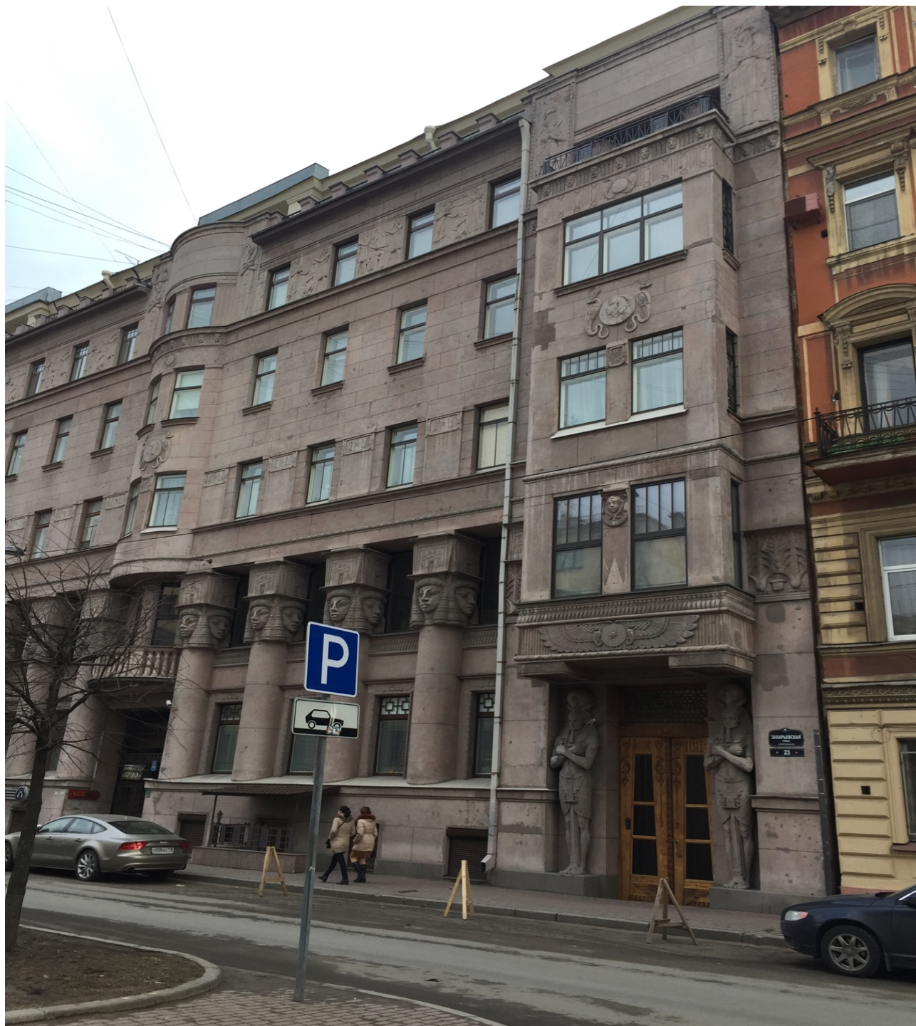
Figure 1. Street view of the “Egyptian House.”
