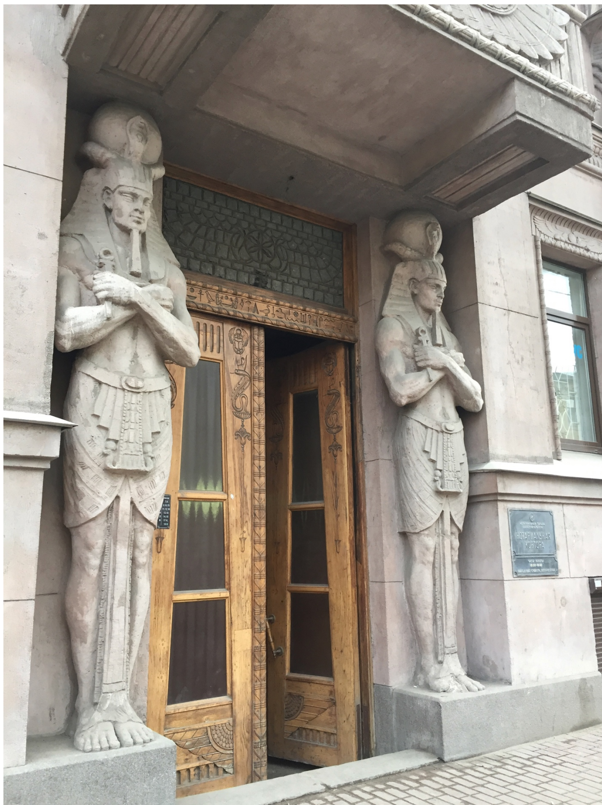
Figure 2. Egyptian house street entrance detail
