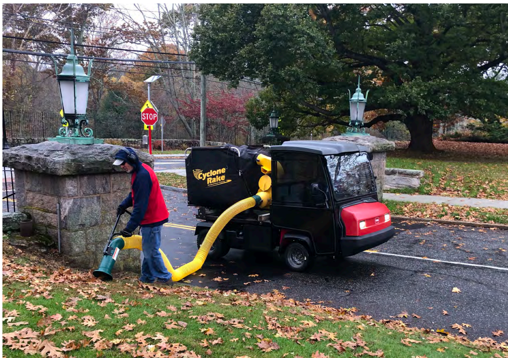
TOP: GROUNDSKEEPER TOM NAZARKO USING AN AIR SPADE TO EXCAVATE SUGAR MAPLE ROOTS IN PREPARATION FOR THE COLLEGE'S FIRST INSTALLATION OF STRUCTURAL SOIL AND A NEW SIDEWALK. STRUCTURAL SOIL IS A COMPACTABLE SUB-GRADE THAT ALLOWS TREE ROOTS TO GROW THROUGH IT.
