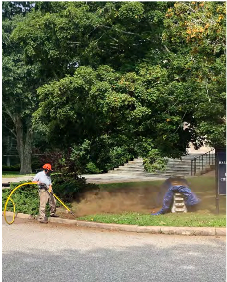
TOP: GROUNDSKEEPER TOM NAZARKO USING AN AIR SPADE TO EXCAVATE SUGAR MAPLE ROOTS IN PREPARATION FOR THE COLLEGE'S FIRST INSTALLATION OF STRUCTURAL SOIL AND A NEW SIDEWALK. STRUCTURAL SOIL IS A COMPACTABLE SUB-GRADE THAT ALLOWS TREE ROOTS TO GROW THROUGH IT.
