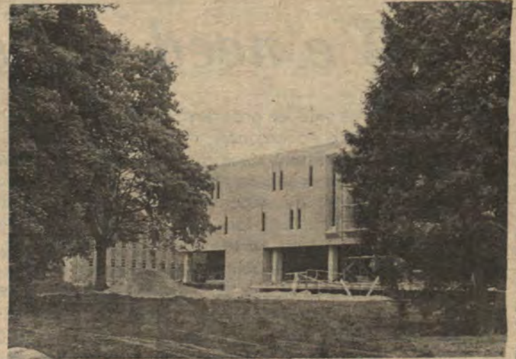
Construction continues on new library.
