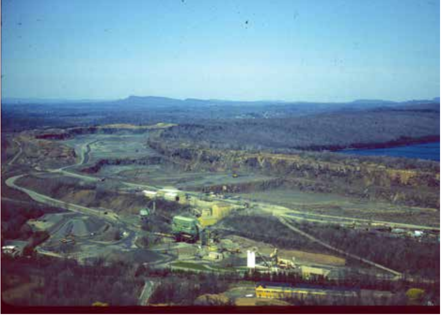
Trap rock quarry in North Branford (CT DEEP)
