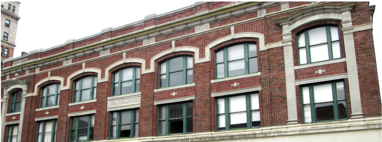
MANWARING BUILDING, 225-237 STATE STREET, NEW LONDON
