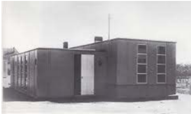
Stahlhaus, 1926 Dessau, Germany Walter Gropius
