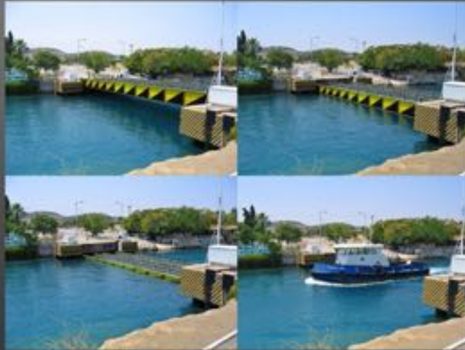
Corinth Canal Bridge, Greece, 1988 *Two submersible bridges designed for the canal, each sinking 26 ft below water level
