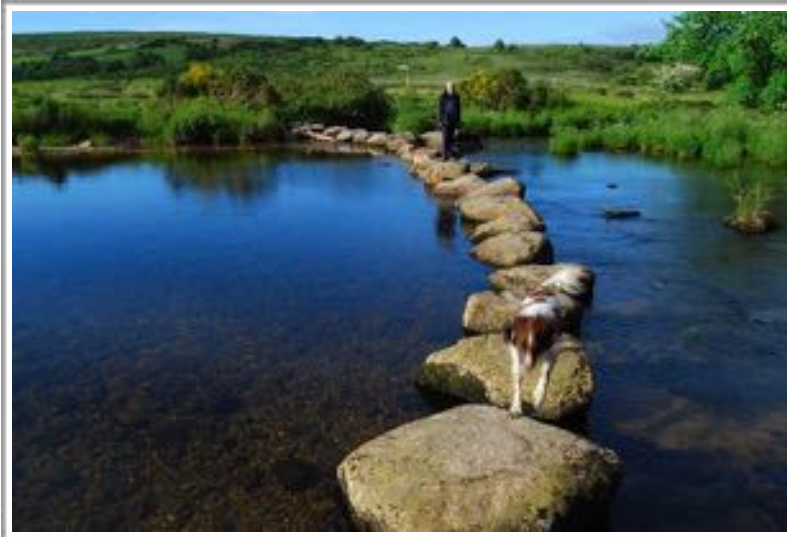
Figure 1.2: Stepping Stone Bridge, Dartmoor, England, 15th century
