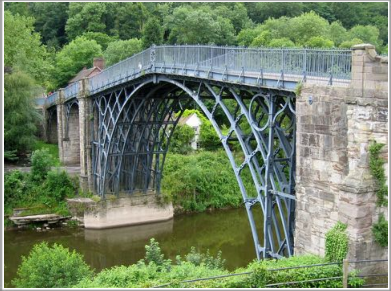
Figure 3.1 The Iron Bridge in Coalbrookdale, Shropshire, England. Although it was “over-designed” the cast iron structure has a beloved delicate design. The stone abutments on either end are massive to counter the outward thrust of the heavy iron arch truss.
