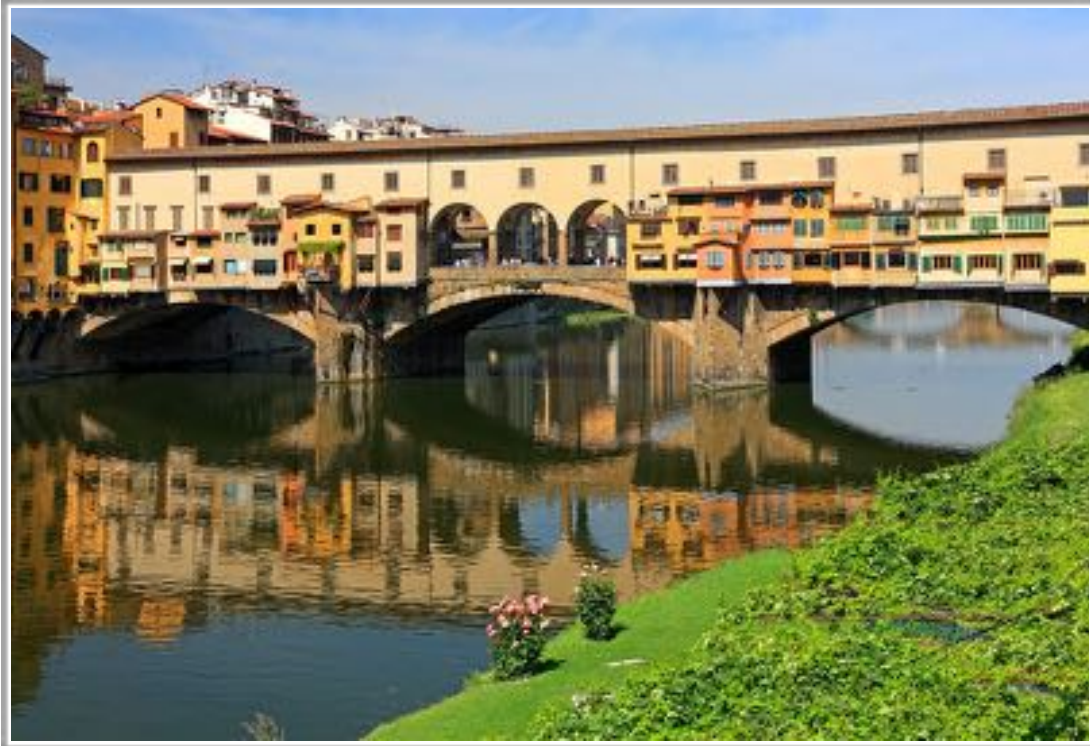
Figure 1.7: Ponte Vecchio, Florence, Italy, 1345; segmental arch bridge, which means it is only part of the circle that is in the arch. The bridge had two predecessors that were destroyed by floods. This is not the first use of buildings on a bridge, the old Tower Bridge in London also used to have buildings on it before it became too weighty for the old bridge.
