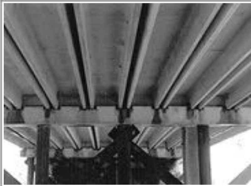
Figures 4.1, 4.2: Example of reinforced concrete channel beams on a construction site and in a finished bridge
