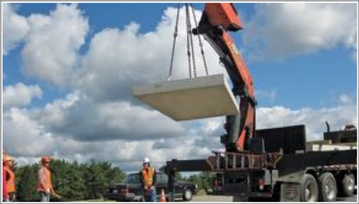
Figure 7.1: Example of reinforced concrete precast slabs on a construction site
