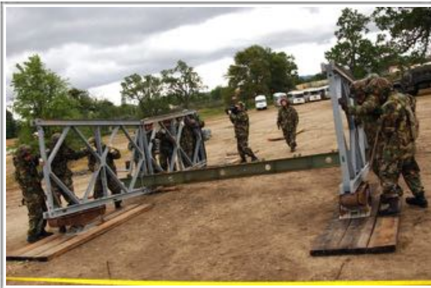
Figures 14.1, 14.2: Examples of Bailey truss bridges
