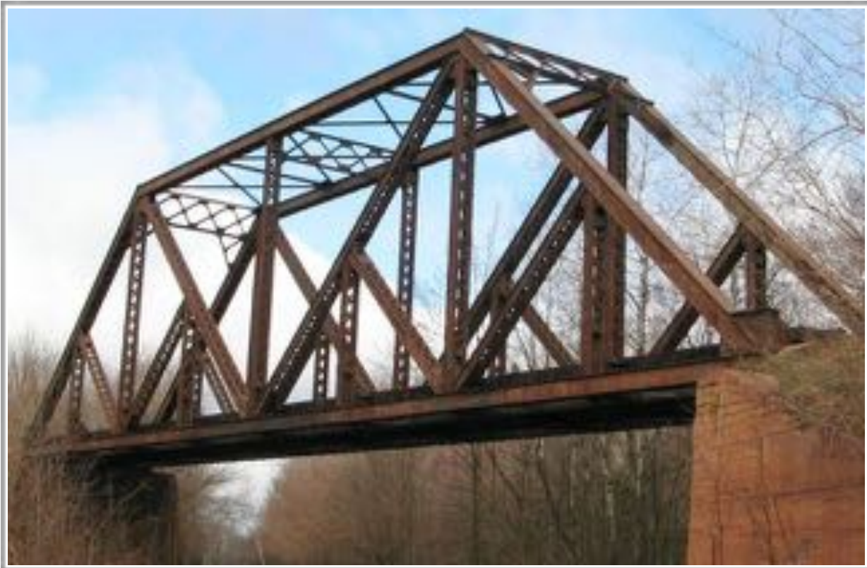
Figure 9.1: Example of a Baltimore truss bridge
