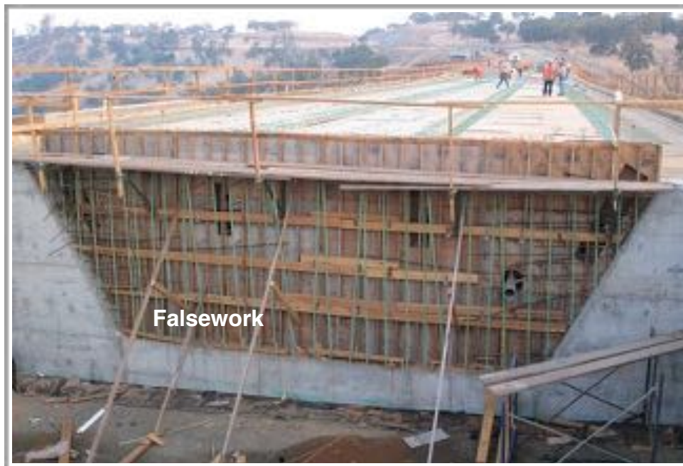
Figure 2.1: Example of a reinforced concrete cast-in-place slab under construction
