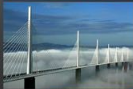
Millau Viaduct (fan)
