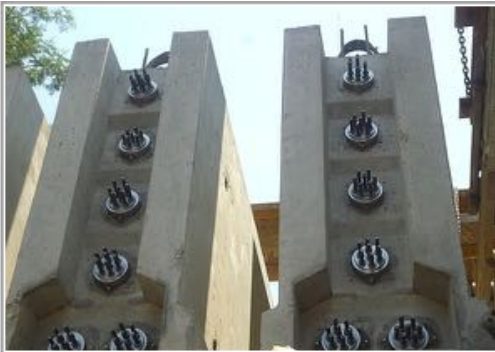
Figures 5.4, 5.5: Examples of pre-stressed and post-tensioned concrete.
