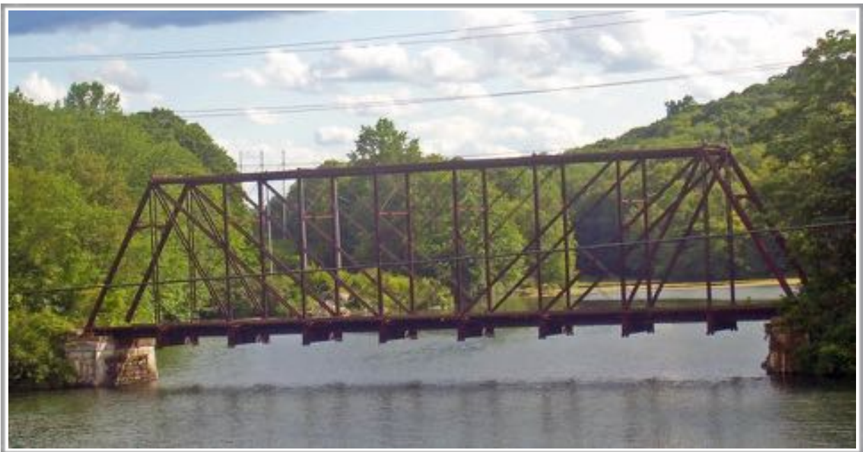
Figure 8.1: Example of a Whipple truss bridge
