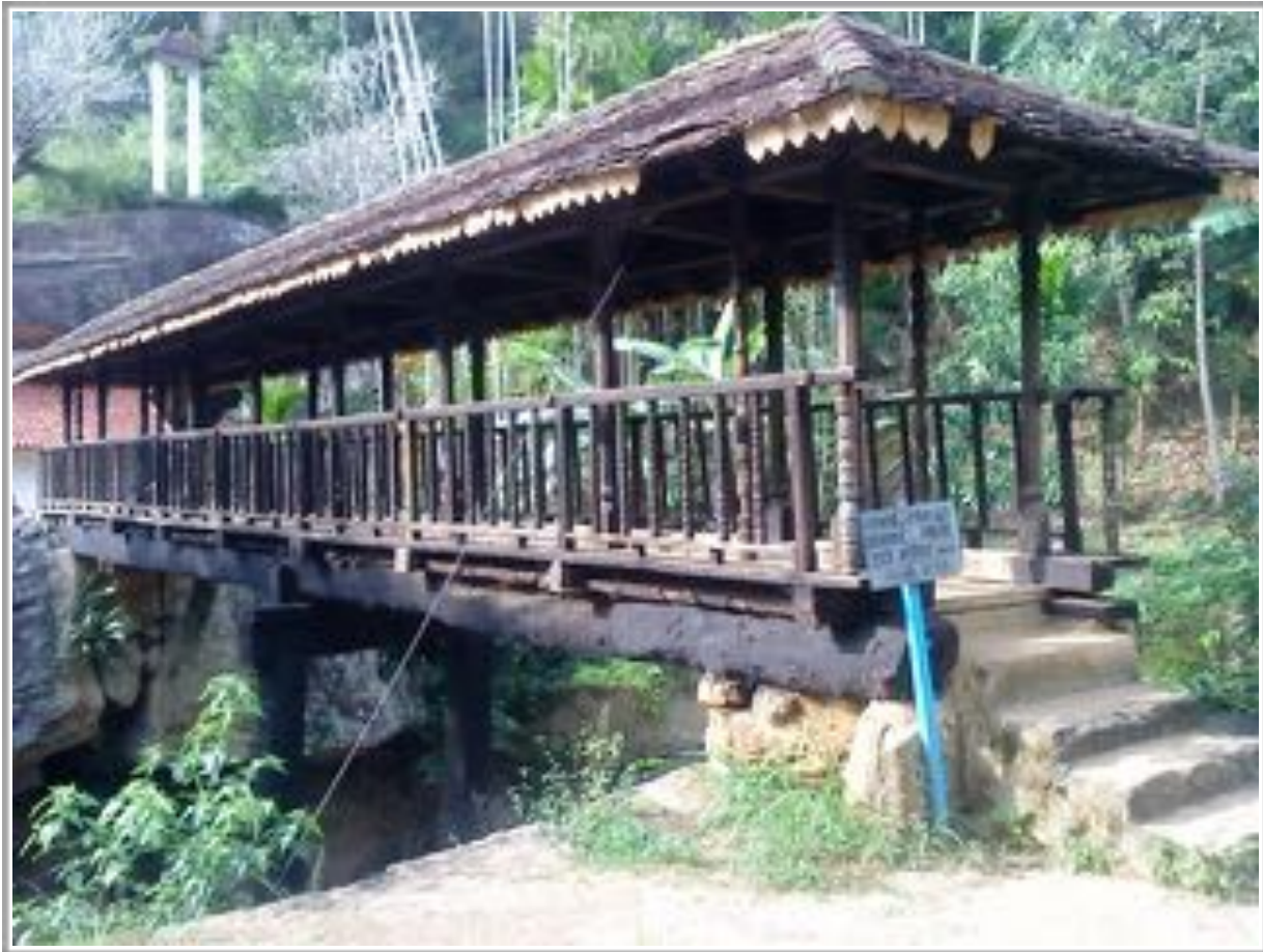
Figure 2.2: The Bogoda Wooden Bridge near Badulla, Sri Lanka, 16 th century. It is one of the oldest continually standing timber bridges in the world. All of its components were constructed from wood including the substructure, decking, roof, roof tiles, balustrade and nails.
