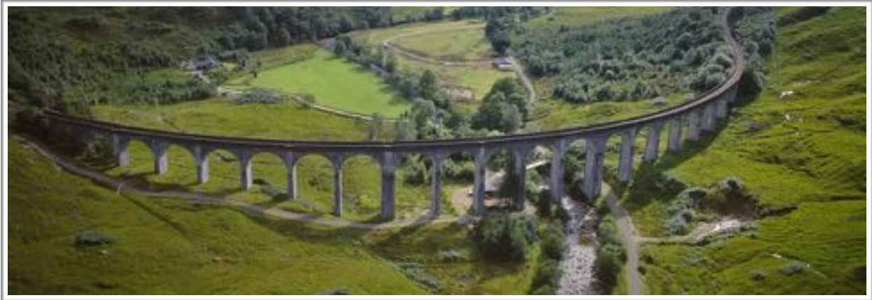
Figure 5.6: The Glenfinnan Railroad Viaduct in Invernessshire, Scotland from 1869. A rare example of a large concrete structure with no reinforcing metal.
