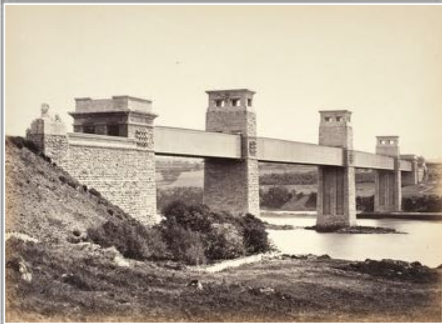
Figures 3.4, 3.5: Robert Stevenson's Britannia Bridge in Anglesey, North Wales from 1850 features wrought iron tubes to handle the long spans. The bridge was a success and remained operational until it was replaced due to a fire in 1970.
