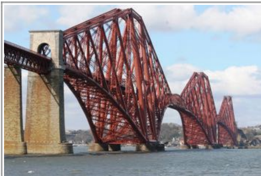
Figures 4.5, 4.6: The Forth Bridge by Sirs John Fowler and Benjamin Baker in Edinburgh, Scotland in 1882. Figure 4.6 is a famous image of the stress test featuring the two designers and an assistant for the project. The test proves that the stress in the men's outstretched arms balance the compression in the lower members, allowing the structure to support a suspended span in the middle.
