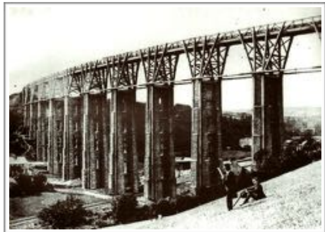
Figures 2.5, 2.6: British Isambard Kingdom Brunel, two examples of his sixty-four wooden railroad viaducts, built between 1849-1864. Due to the rising railway industry there was a new need for bridges that had to be met quickly. Brunel worked strictly in wood to create 64 viaducts for the South Devon, West Cornwall and Cornwall Railways.
