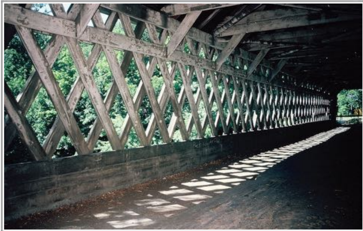
Figure 4.1: Example of a Lattice truss bridge
