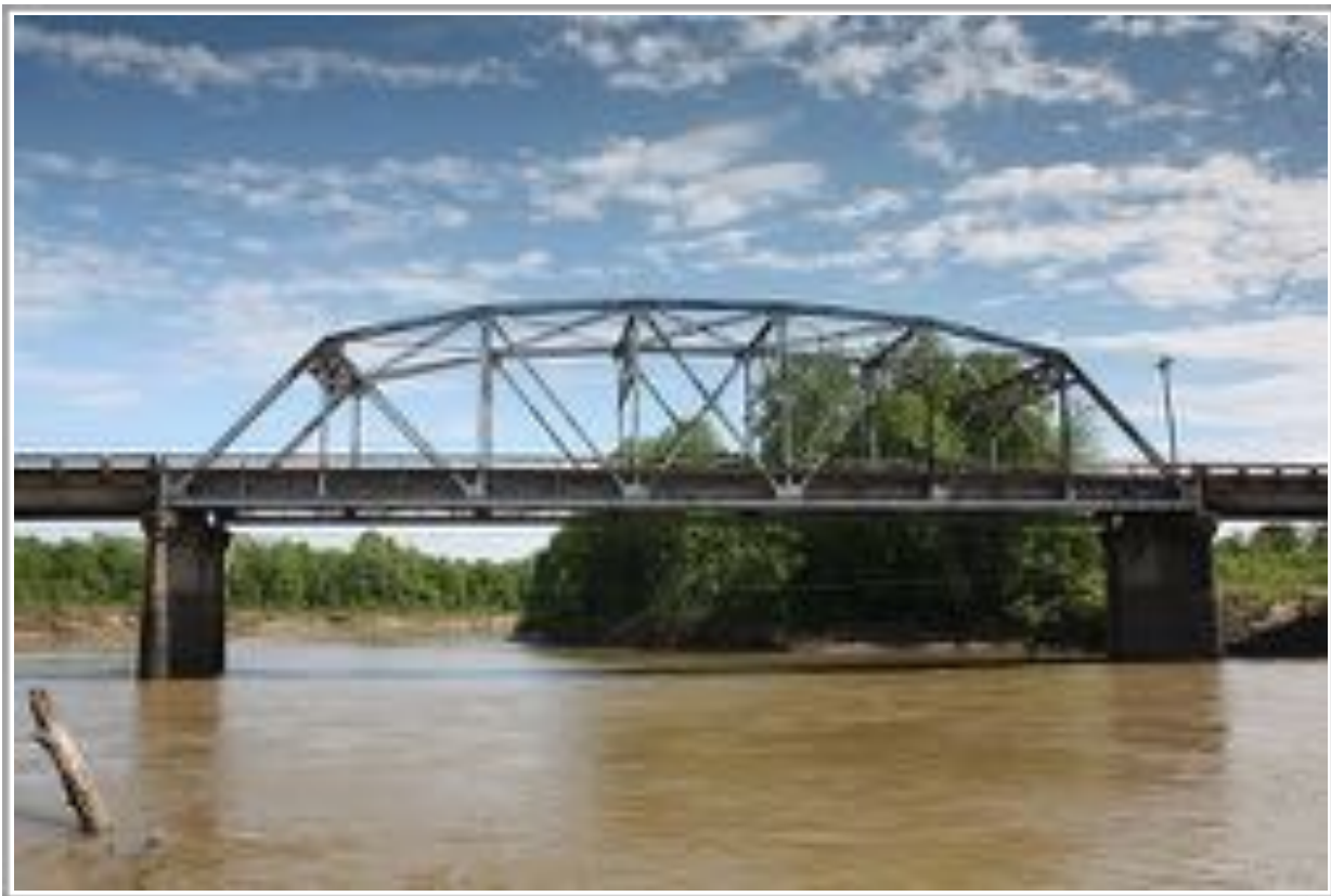
Figure 11.1: Example of a Parker truss bridge
