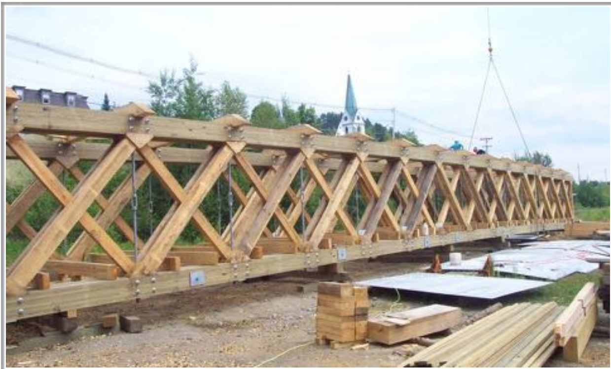
Figure 3.1: Example of a Howe truss bridge
