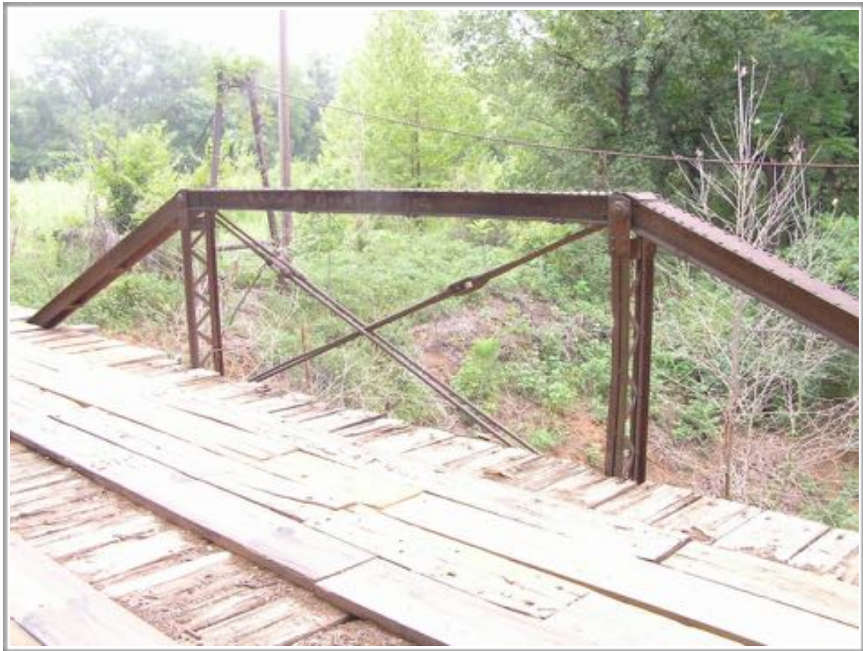
Figure 2.1: Example of a queen post truss bridge
