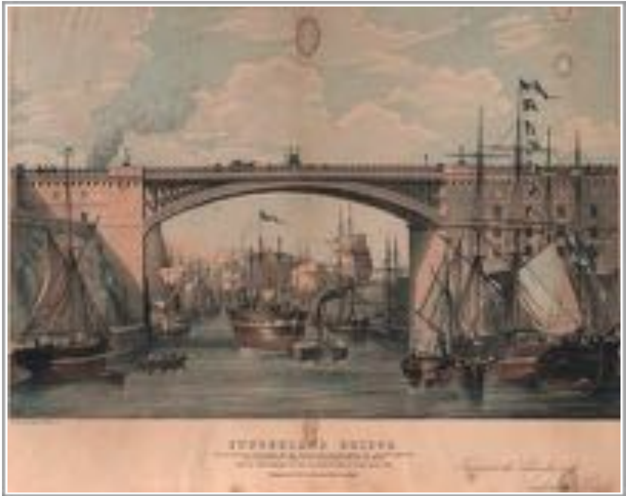
Figure 3.2: Thomas Wilson's Sunderland Bridge in the North of England, built in 1793-96, took an evolutionary step in creating a segmental design with twice the span of any previous cast iron bridge. Again, the abutments on the banks are large to handle the weight of the iron span.
