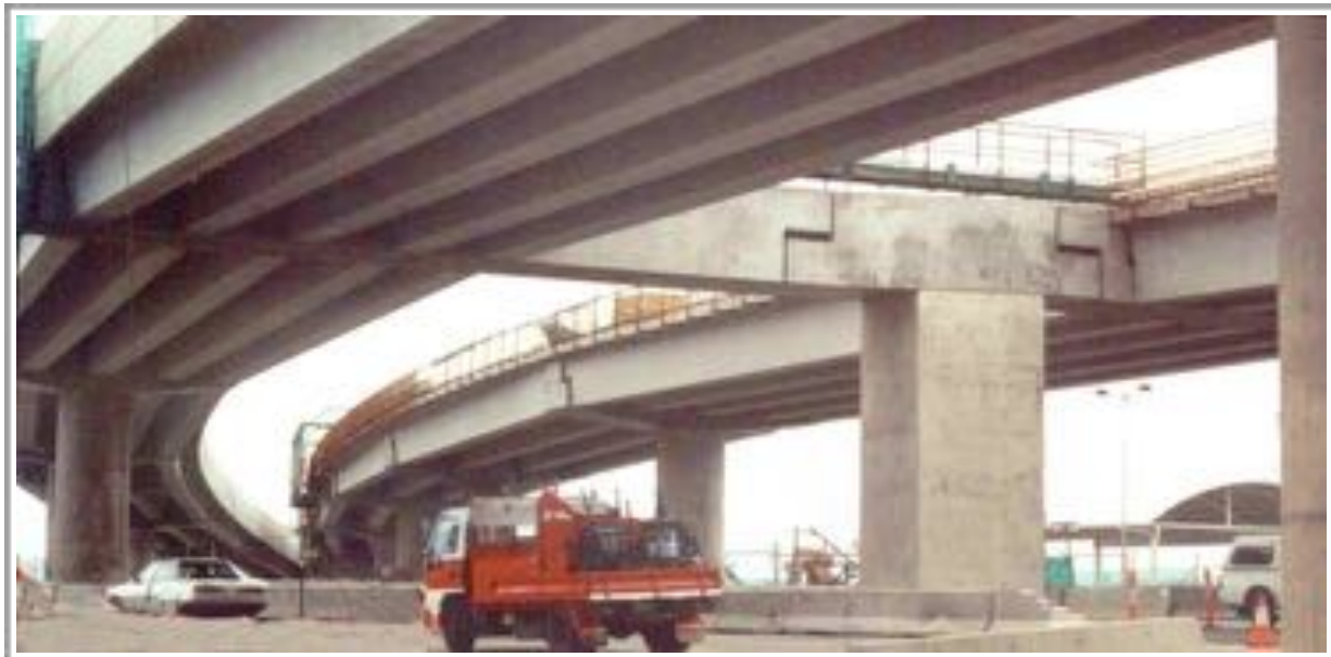
Figure 5.1: Example of a reinforced concrete girder bridge
