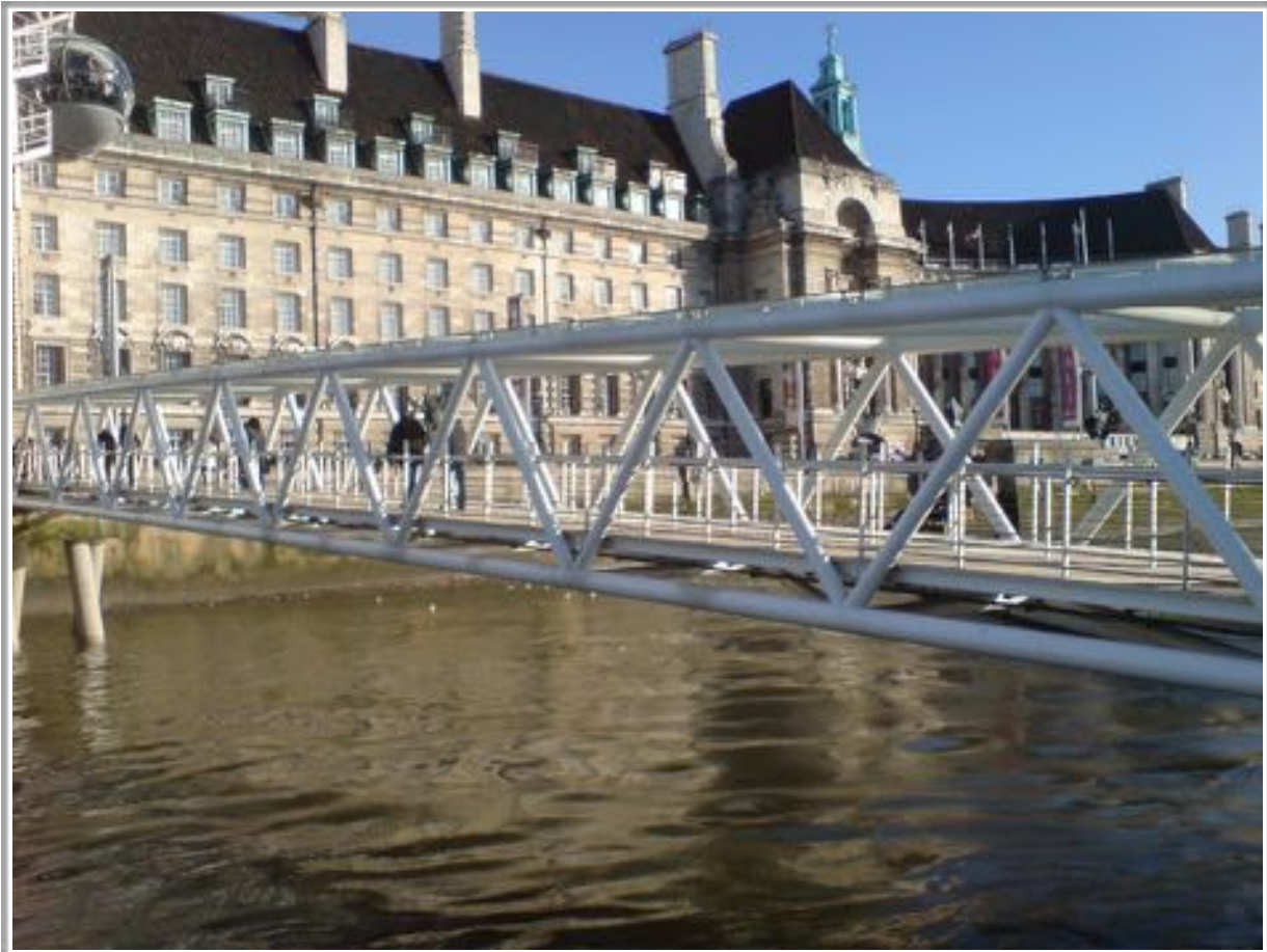
Figure 12.1: Example of a Warren truss bridge
