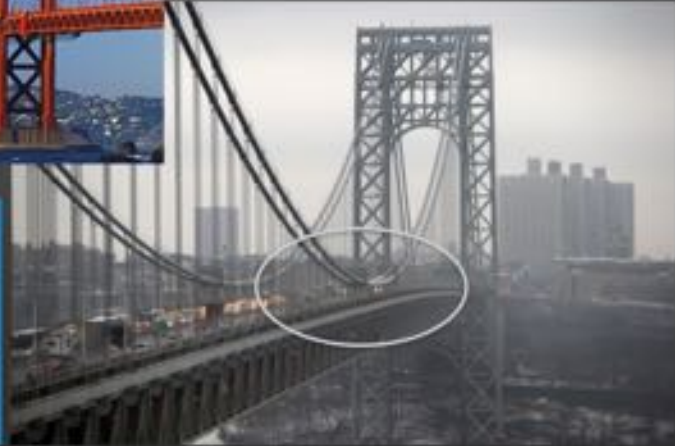
George Washington Bridge *Fun Fact: Originally the towers were to be clad in stone but they ran out of money. The basic structural design was deemed aesthetically pleasing in itself and remains today
