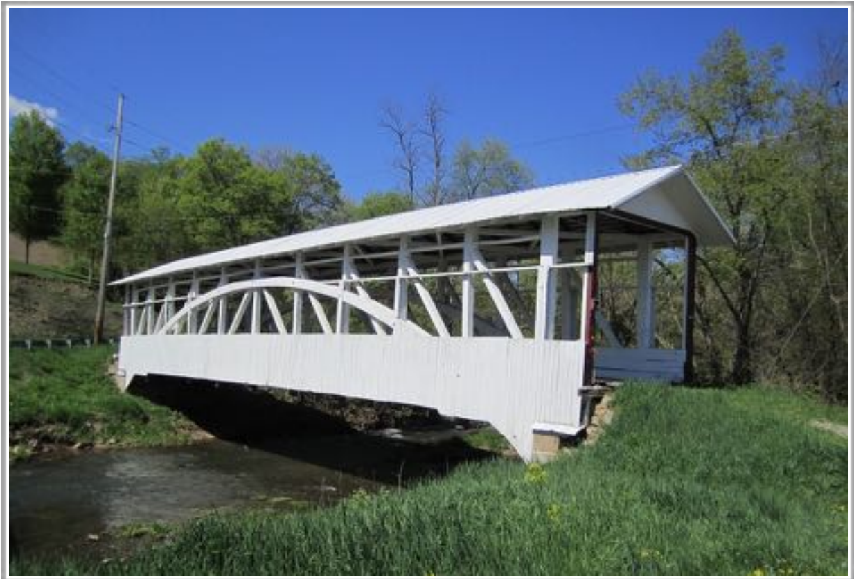
Figure 5.1: Example of a Burr truss bridge
