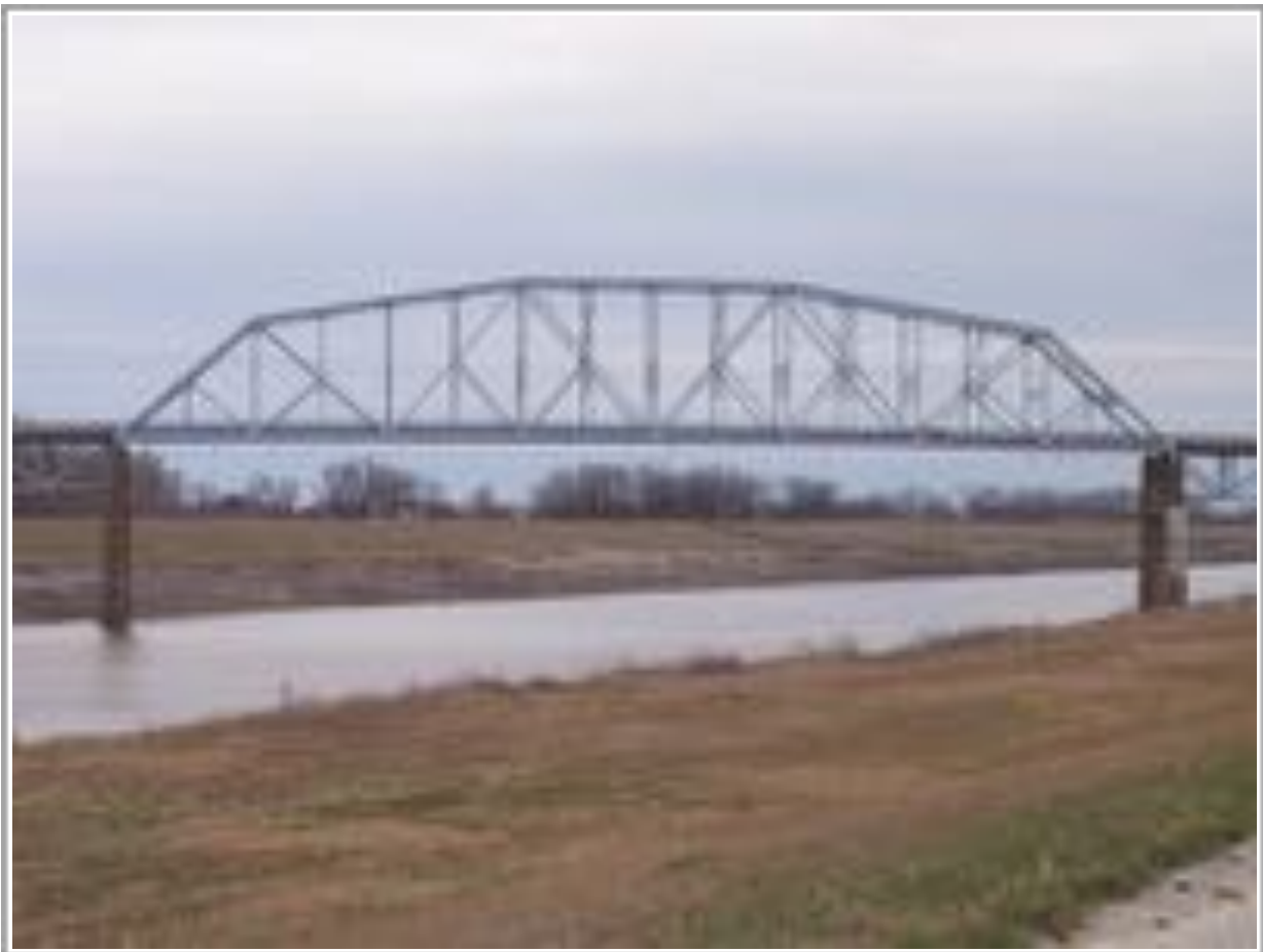
Figure 10.1: Example of a Pennsylvania truss bridge
