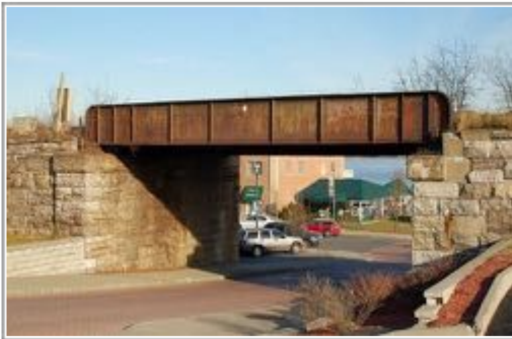
Figures 11.1: Example of metal built-up girder bridges
