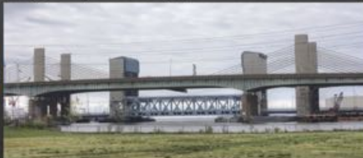
I-95 Northbound bridge, New Haven, CT. First extradose bridge in the US
