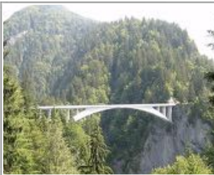
Figure 5.8 Robert Maillart's Salginatobel Bridge in Schiers, Switzerland in 1930. The thin and simple 250-foot arch soars 1,000 feet above the valley below, making the bridge a landmark in concrete history. Bridge expert David Billington applauds Maillart's design and vision stating he "was the first engineer to sense that the full expression in concrete structures could be efficient (safe performance with minimum materials), economical (accountable to the public welfare or private industry with competitive costs), and elegant all in the same construction."
