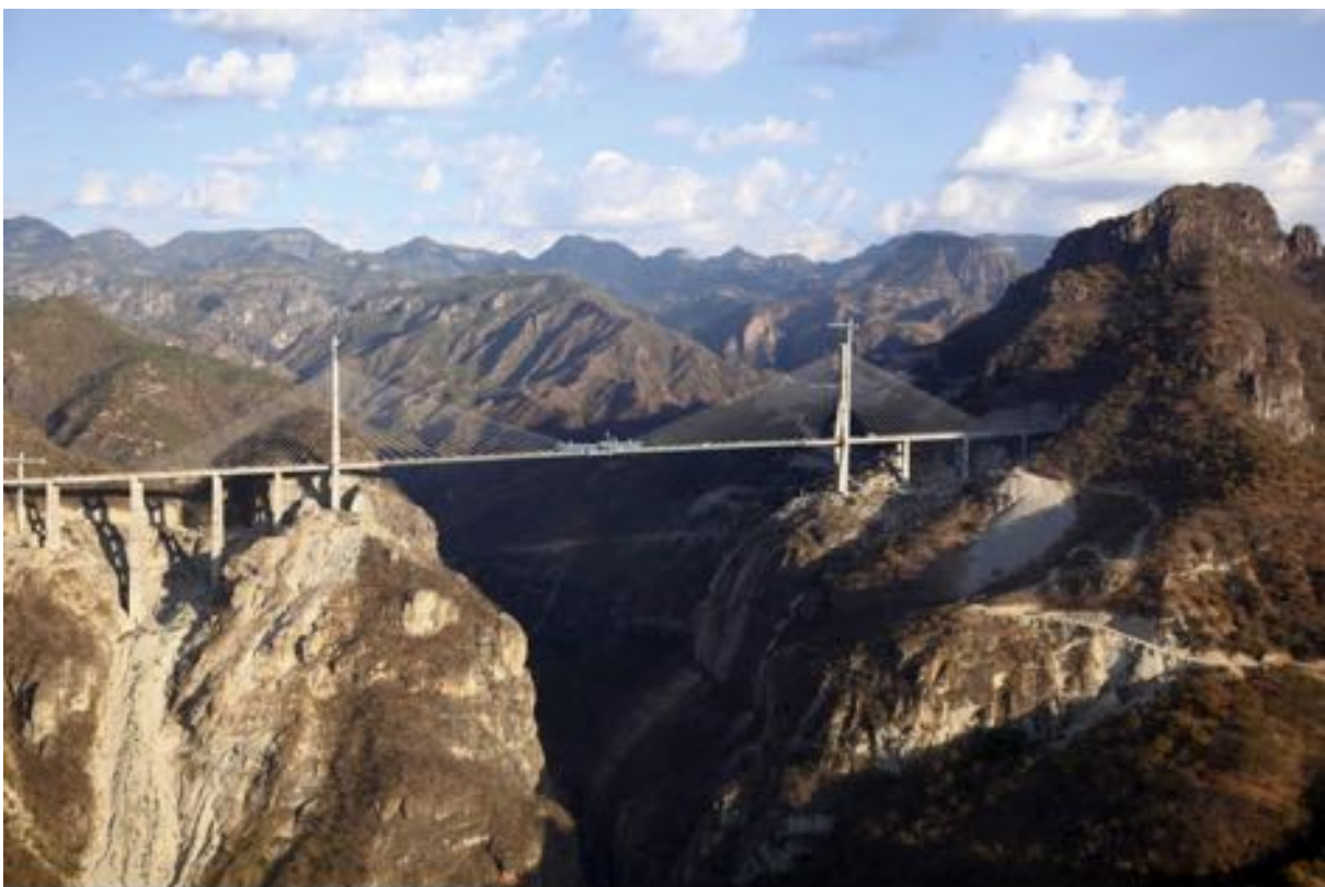
Baluarte Bridge, Durango, Mexico, 2008
