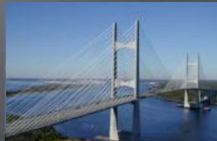
Dame Point River Bridge (harp)
