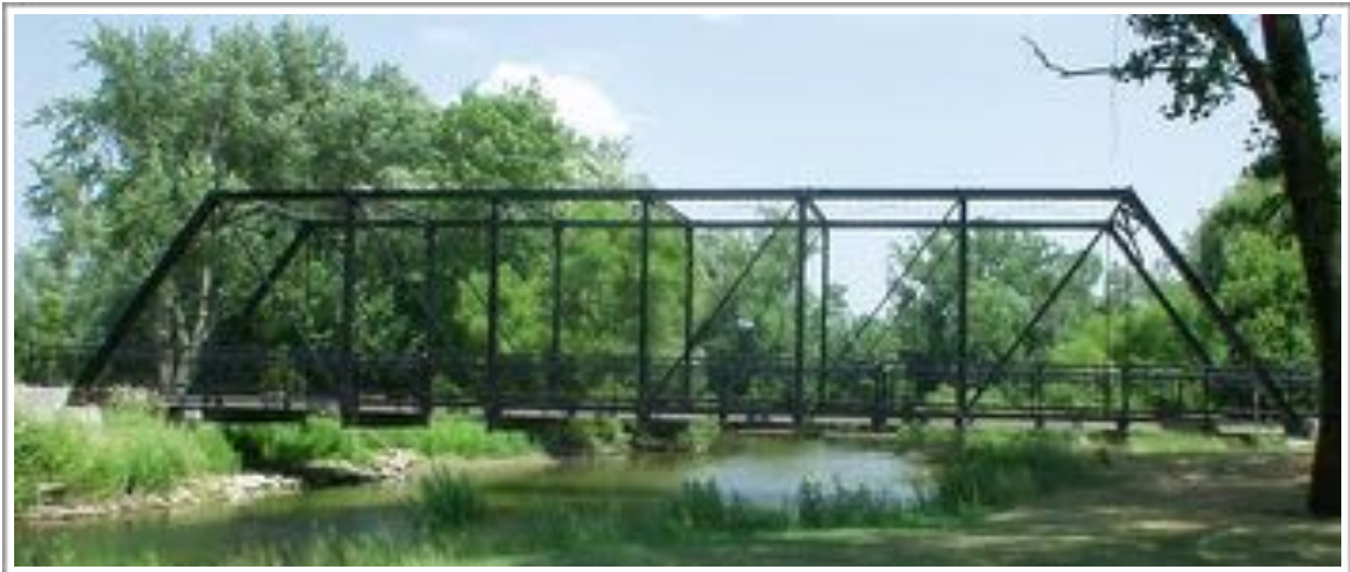
Figure 7.1: Example of a Pratt truss bridge
