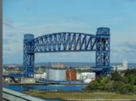
Arthur Kill Vertical Lift Bridge, Elizabethport, NJ and Staten Island, NY, 1959 *longest lift span in the world: 558 ft truss
