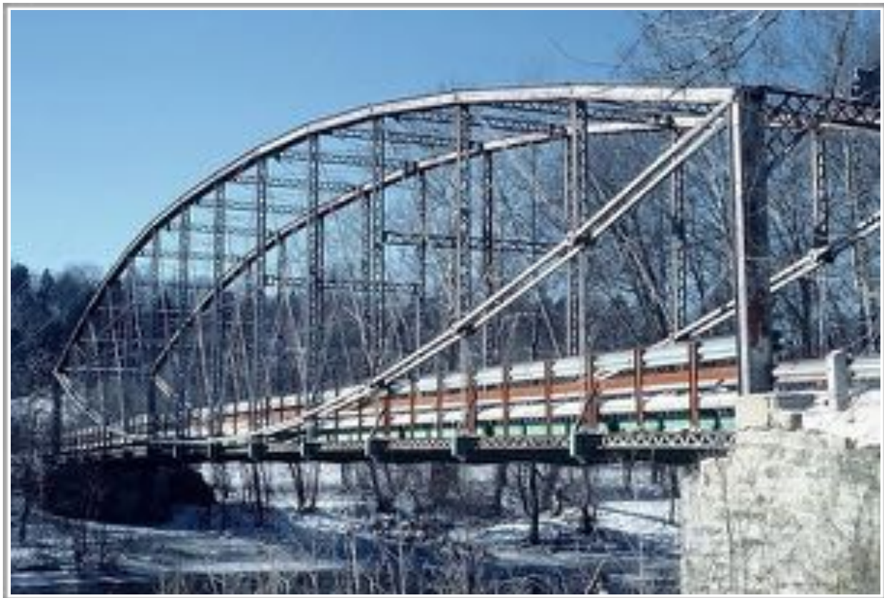
Figure 13.1: Example of a Lenticular truss bridge
