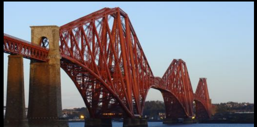
The Forth Bridge, Edinburgh, Scotland, 1882
