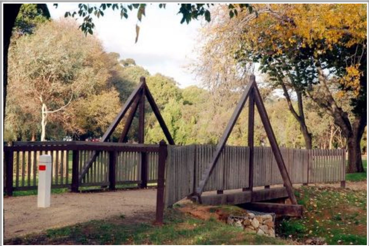
Figure 1.1: Example of a king post truss bridge
