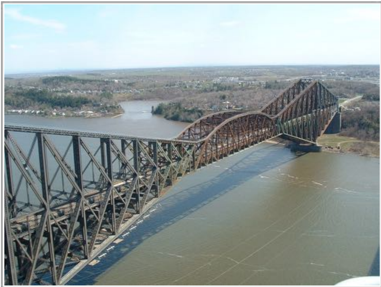
Figure 15.1: Example of a cantilevered truss bridge
