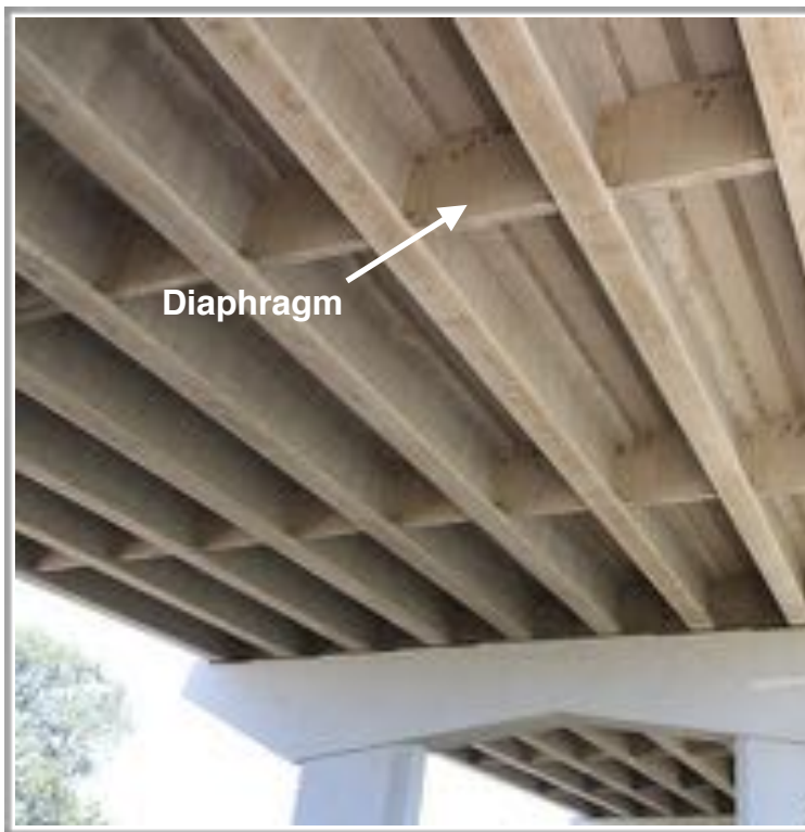
Figures 8.1, 8.2: Examples of reinforced concrete I-beams on a construction site and in a finished bridge. Also, a visual example of a diaphragm, a common secondary support in bridges.
