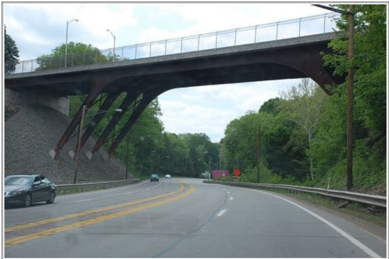
Figure 12.1: Example of a steel rigid frame bridge
