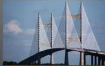
Dame Point River Bridge (harp)
