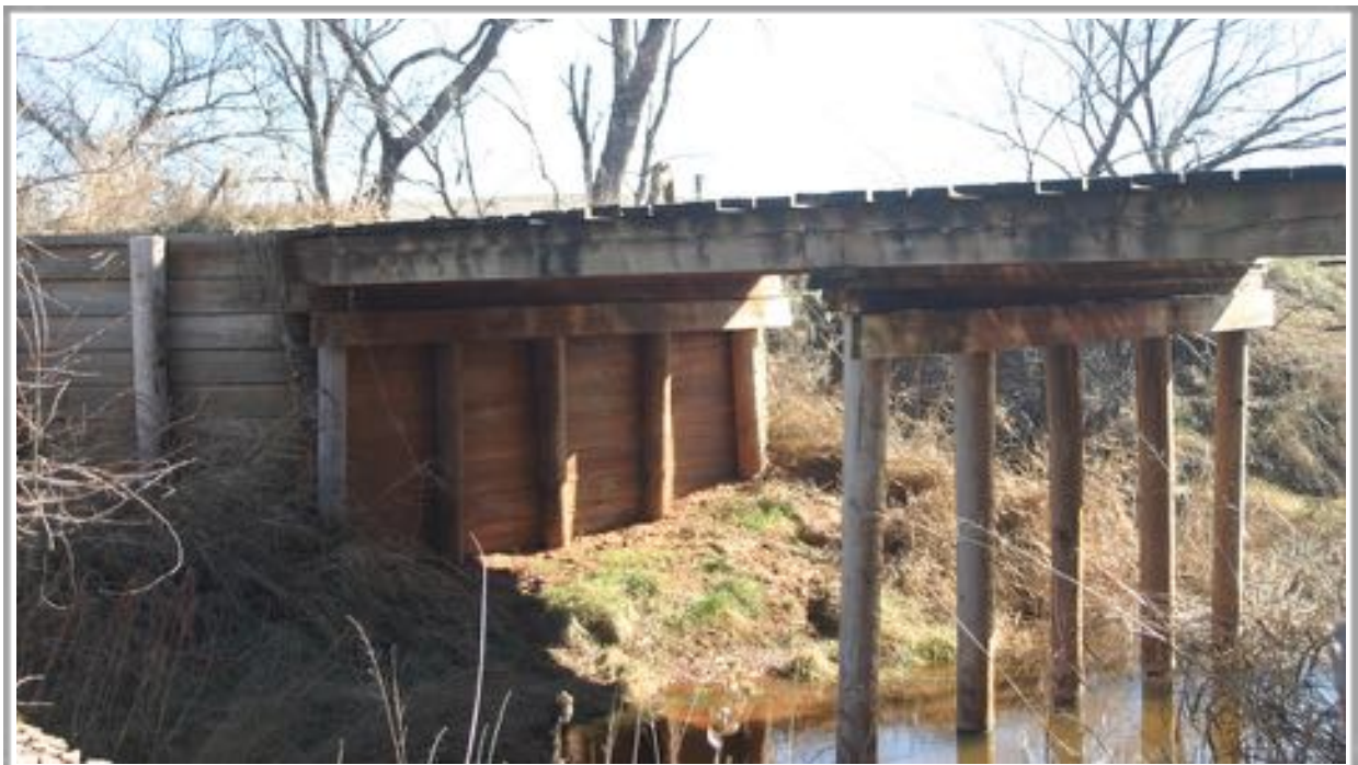
Figure 1.1: Example of a timber stringer bridge
