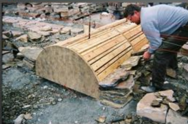
Temporary wooden falsework for construction
